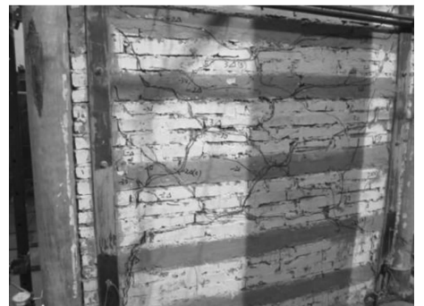
图8 试件 KJ-3 破坏形态 Fig. 8 Failure mode of specimen KJ-3
