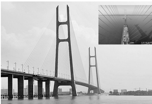
图8 某长江公路大桥施工及成桥状态 Fig. 8 The construction and finished bridge state in certain yangtze river highway bridge
