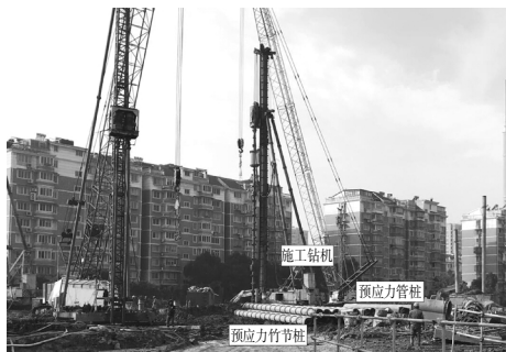
图 2 静钻根植桩现场施工图 Fig.2 Photograph of pre-bored grouted planted pile installation process
