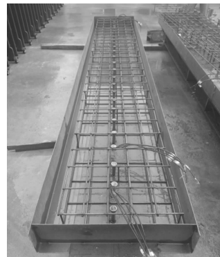
图 4 FBFT-4 模板及配筋 Fig. 4 Formwork and bars of FBFT-4
