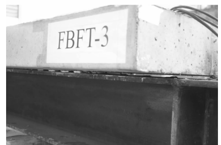
图7 混凝土板掀起 Fig.7 Uplifting of concrete slabs
